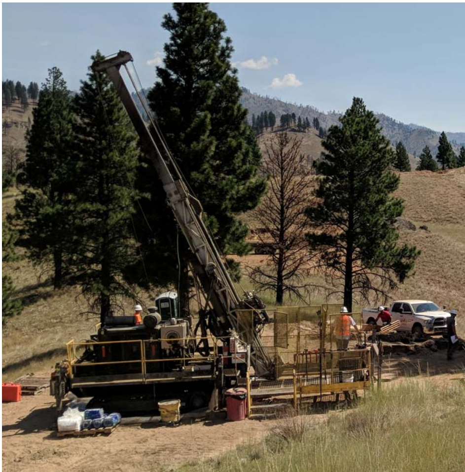
Photo showing the drilling rig set up to drill the Company’s first hole at the Colson Cobalt-Copper Project, Idaho
