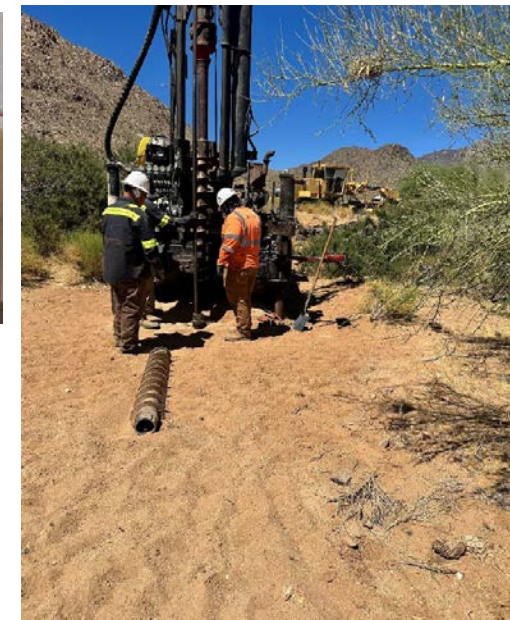
Surface Geotechnical Investigation – Cascade Drilling
