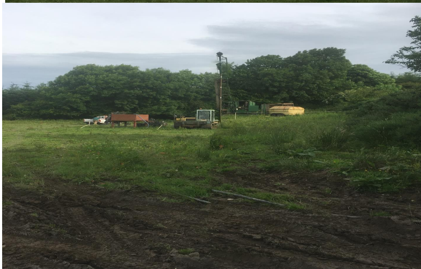
Two Drill mask up and drilling at Keel Zinc Project
