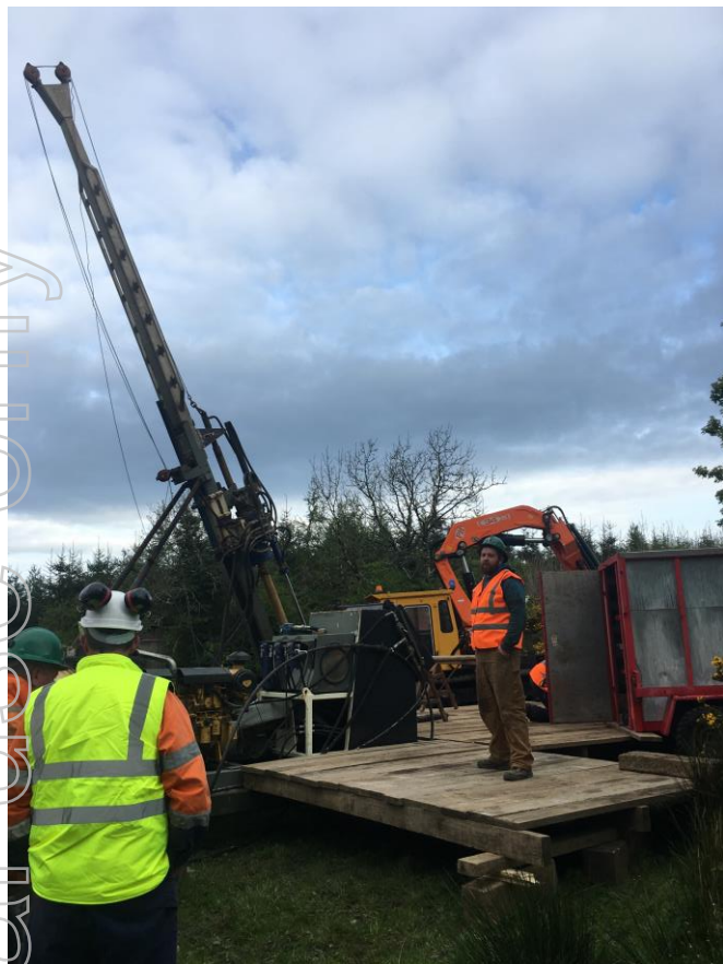
Figure 1 Drill Rig Platform
